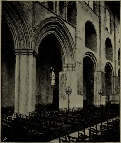
NAVE, NORTH SIDE.
